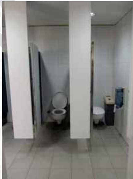
CONTEMPORARY WC FITOUT.
