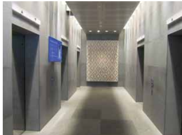
LOW RISE LIFT LOBBY WITH NEW CLADDING
