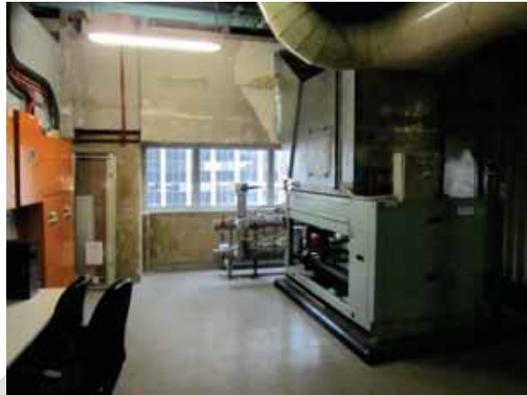
GENERAL PLANT VIEW
