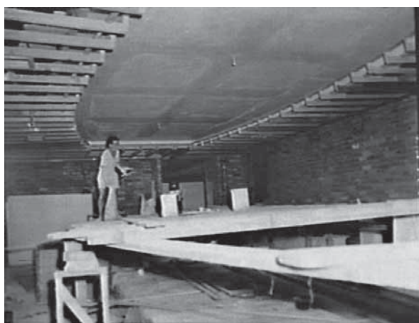
THE BOARDROOM UNDER CONSTRUCTION
