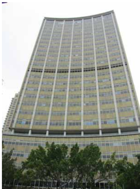
NORTHERN GLASS CURTAIN WALL
