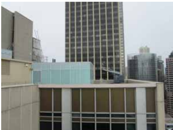
VIEW SOUTH SHOWING C.2000 ADDITIONS (WESTERN SIDE)
