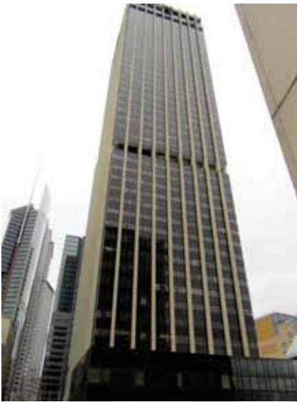
VIEW SOUTH TO 50 BRIDGE STREET (AMP CENTRE)
