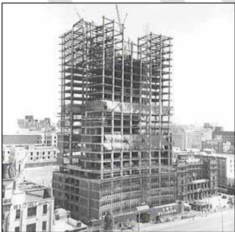
FIGURE 52 – THE AMP BUILDING DURING CONSTRUCTION, 1961
