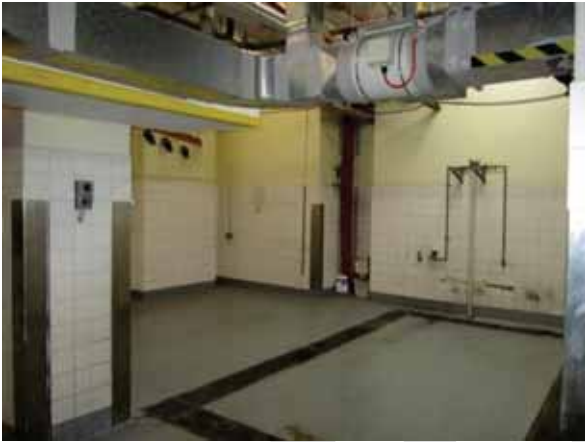
ORIGINAL CARWASH FACILITY
