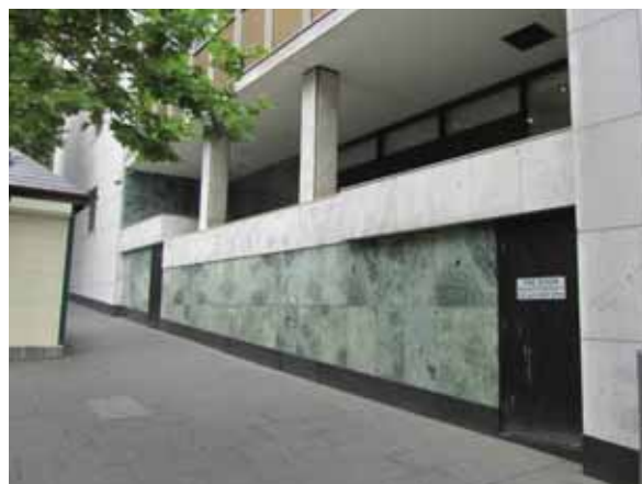
THE FORMER PHILLIP STREET ENTRY (NOW ENCLOSED).
