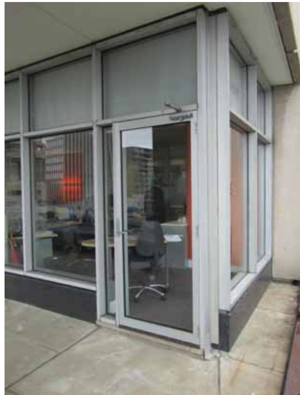
NORTH WESTERN CORNER ACCESS TO THE TERRACE.
