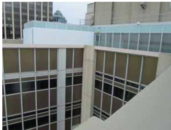
VIEW SOUTH SHOWING C.2000 ADDITIONS (EASTERN SIDE)
